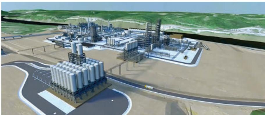
This artist's rendering shows Shell Chemical Appalachia LLC's plan for a petrochemical complex to be built northwest of Pittsburgh that will produce ethylene and polyethylene from Marcellus and Utica shale ethane. Image from Shell.
